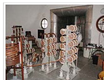
Power ceramic capacitors in a radio-frequency transmitter station
