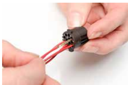
Step 4 - Push wire into insert
