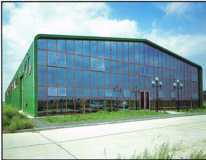
Terminal Box factory
