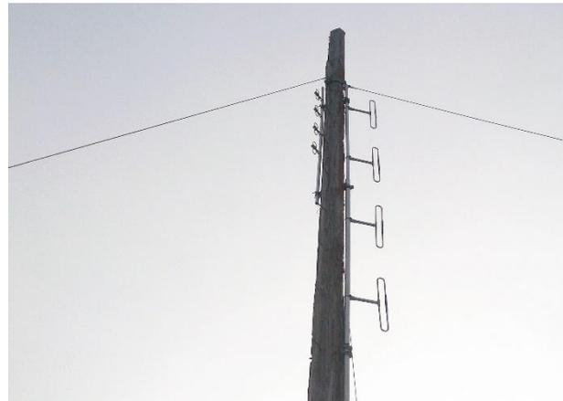
With good engineering, this can be done in such a way that the services do not interfere with each other and without degradation of antenna performance. The picture shows the main VHF stack, which consists of two bays. Two dipoles are used for transmit and two dipoles for receive. The 7075, WREMO and Surf repeaters all share the receive pair.
