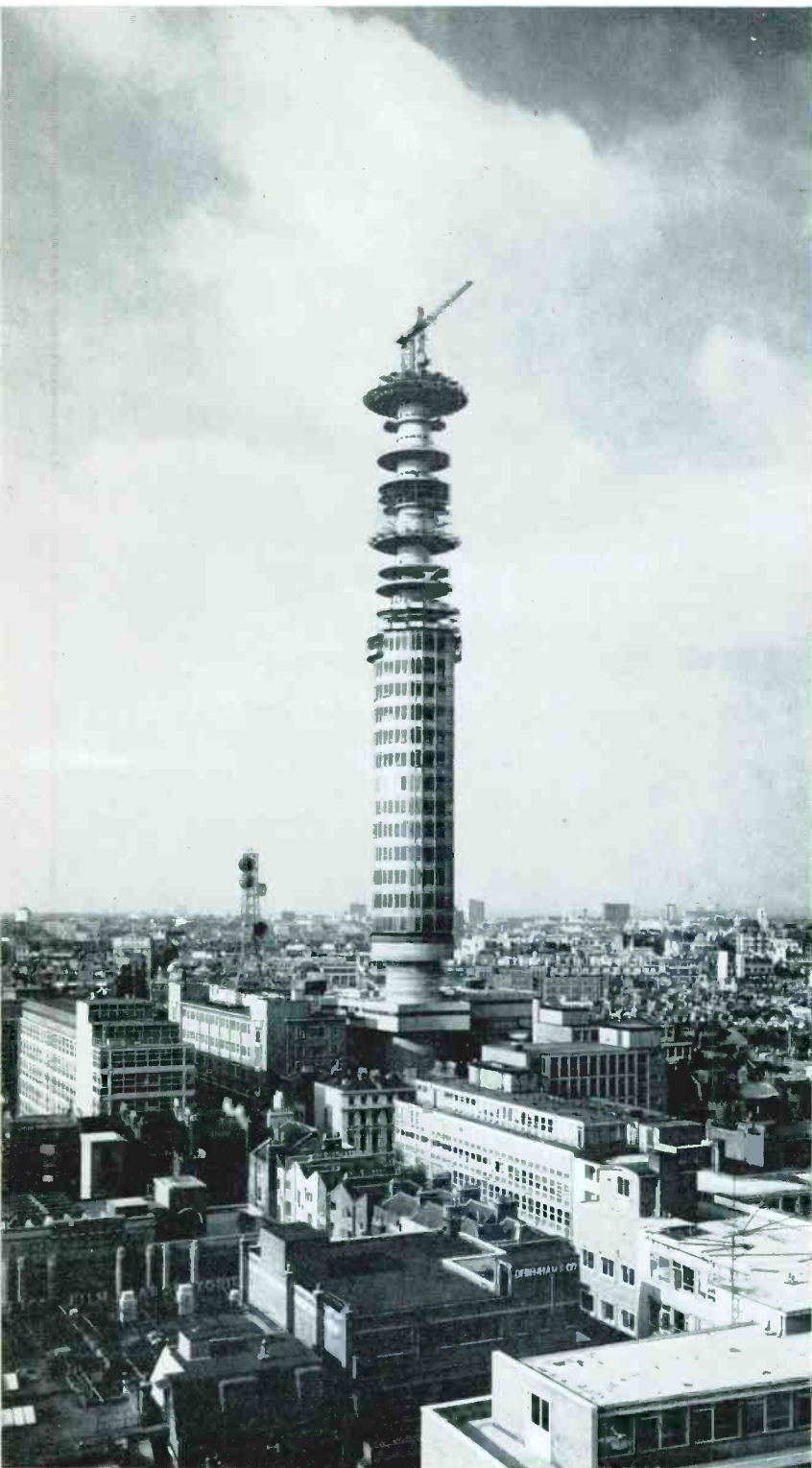
Museum telephone exchange radio tower in the course of construction in the Tottenham Court Road area of London. To minimize the possibility of intermodulation distortion between channels, due to imperfections in the waveguide runs, the radio receivers will be housed immediately beneath the aerial galleries
