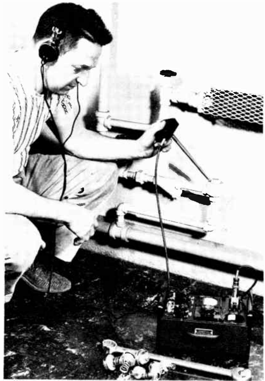
Figure 12-6. Checking a steam trap with vibration-measuring equipment.
