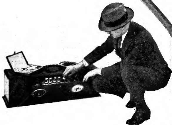
THE upper cut shows John B. Brennan, Technical Editor of RADIO BROADCAST, substituting Brightson True Blue Tubes in the Radiola super-heterodyne, so that it may be operated from the automobile storage battery. The center photograph shows the space left in the battery compartment of the "super" when the dry cell A batteries are removed
