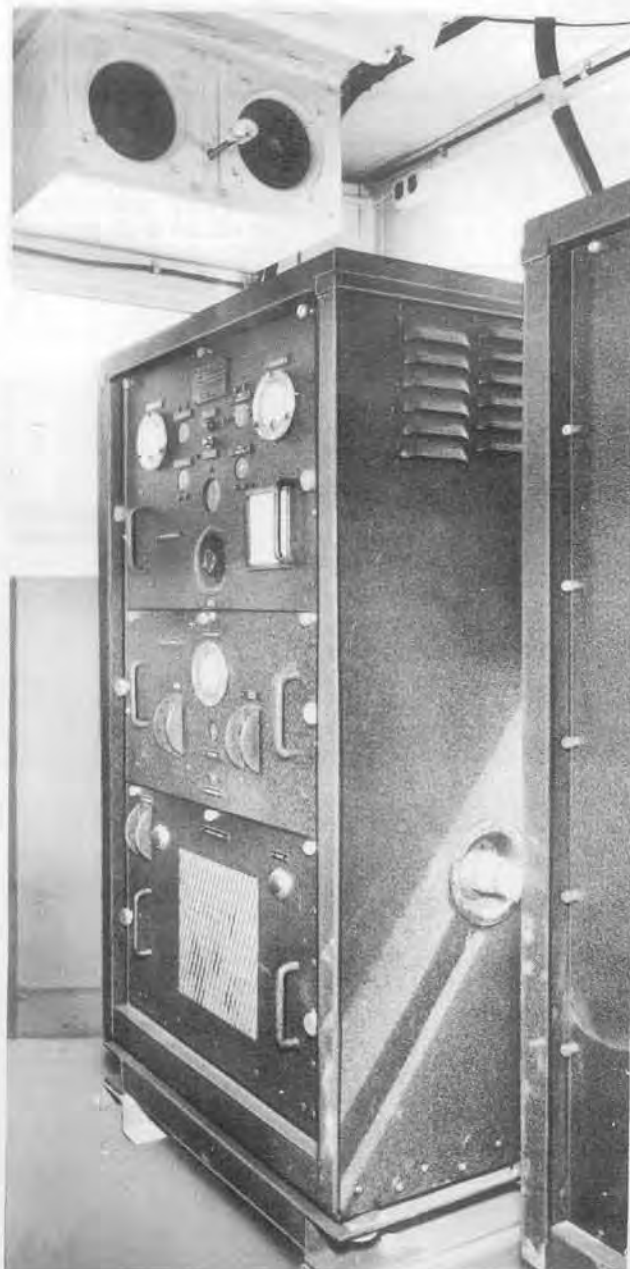
Radio Transmitter BC-751 installed in truck.
