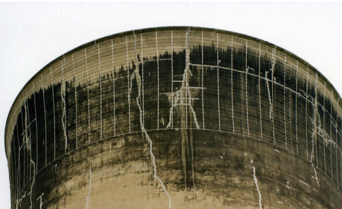
Cooling Tower Repair
