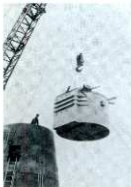
Inset: Positioner Being Lifted Into Position
