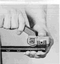
**5.** Set the blade of the cable sheath cutter so that it is located in the space between the conductor core units and the laminated cable sheath. Make the longitudinal cut by holding the cable against the serrated gripper and pressing down the hand lever.
