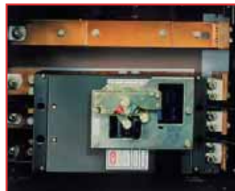
MCCB Rotary Handle Mechanism
