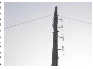
With good engineering, this can be done in such a way that the services do not interfere with each other and without degradation of antenna performance. The picture shows the main VHF stack, which consists of two bays. Two diploes are used for transmit and two diploes for receive. The 7075, WREMO and Surf repeaters all share the receive pair.
