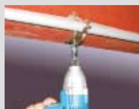
Installing piping or wiring supports
