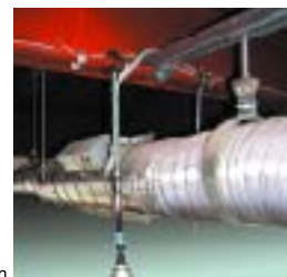
Hanger bolts for duct installation
