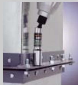
Tightening of duct coupling
