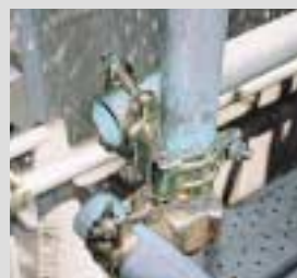
Tightening of step clamp
