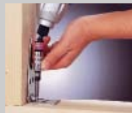
Installing tension and angle brackets
