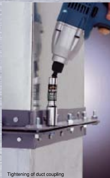
Tightening of duct coupling
