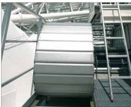
Steel cable carriers on a scissored coil lift Photographs: SKO Steiner GmbH
